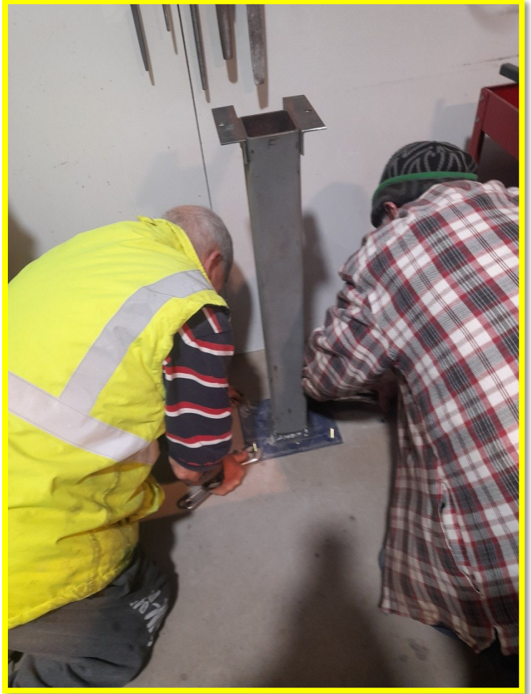
Bottoms up Ian A & Trevor A installing a heavy duty post for a grinder
