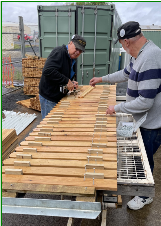
Peter Ha & Peter He assembling panels using spacers on the pickets in an alignment jig
