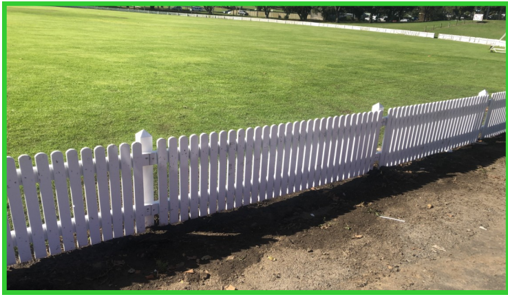
New fence panels are being installed at Frew Park
